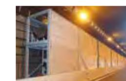
Pipe conveyor belt installed along expressway shoulder
